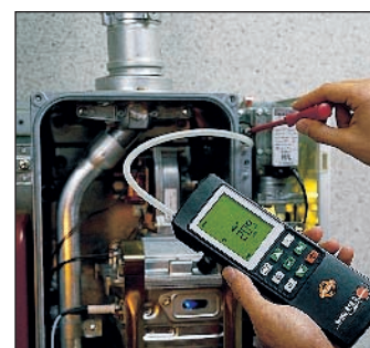
Differential pressure measurement on heating units
