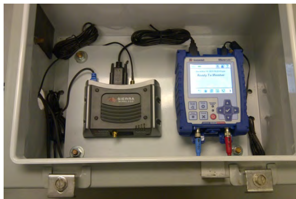
Mounting Panel Installed in the Enclosure
