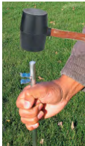
Hard Ground Installation
