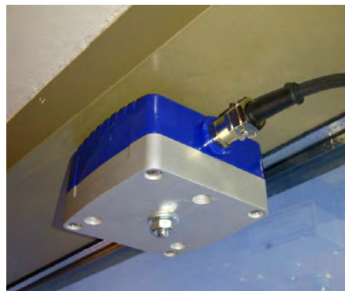
Geophone Mounted to the Ceiling
