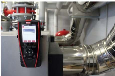
Climatic conditions measurement
