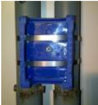
Micromate Attached with Metal Straps
