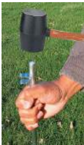
Hard Ground Installation
